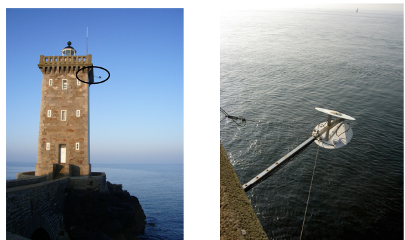
Figure 4 - Oceanpal antennas deployed on top of the Kermorvan lighthouse. OPIF campaign.
